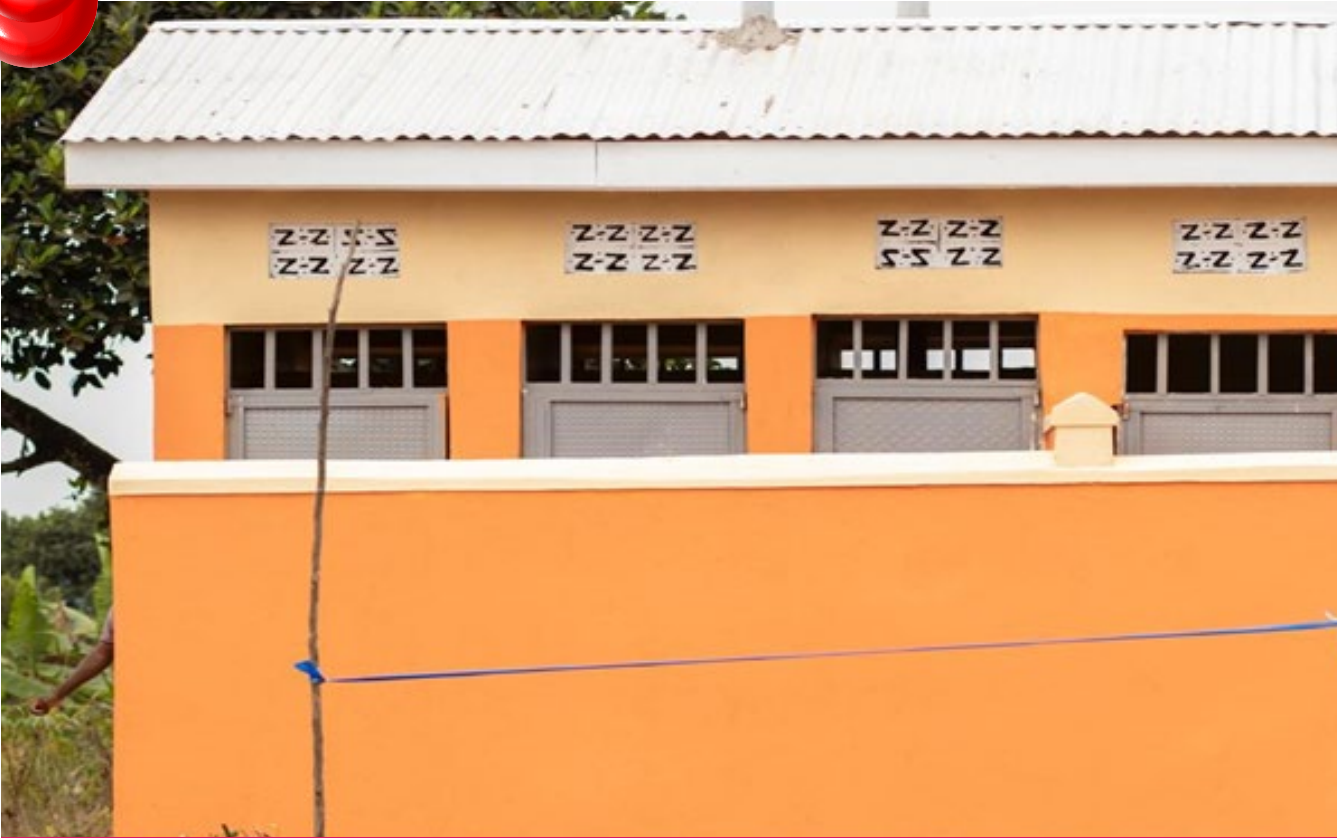
Handover project of a pit latrine in Masaka district at St. Micheal primary school by the Rotaract Club of Kampala the Core led by President Arinda Sonia on the 16th August,2025
